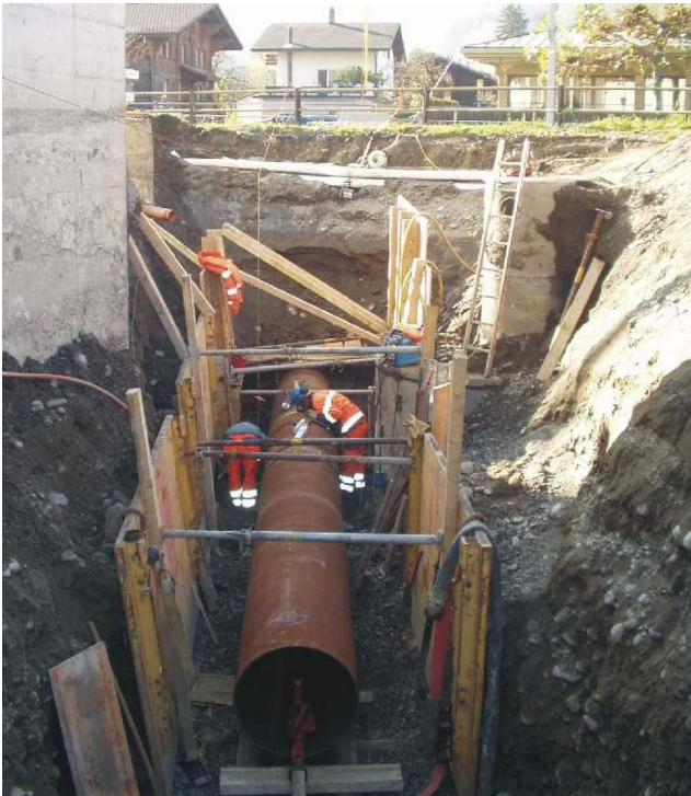
The steel pipe Ø 800 mm (32 inch) is adjusted exactly in the ramming pit.
