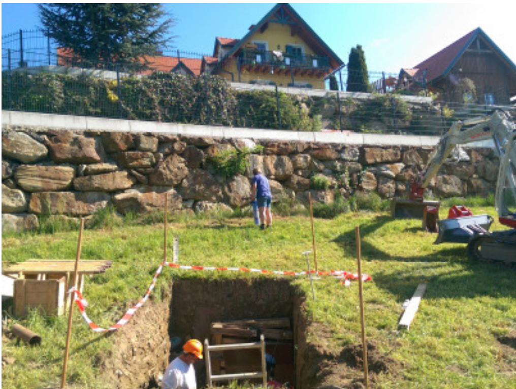
Pic. 1: The non-disruptive crossing of two staggered stone walls and the adjacent forecourt.
