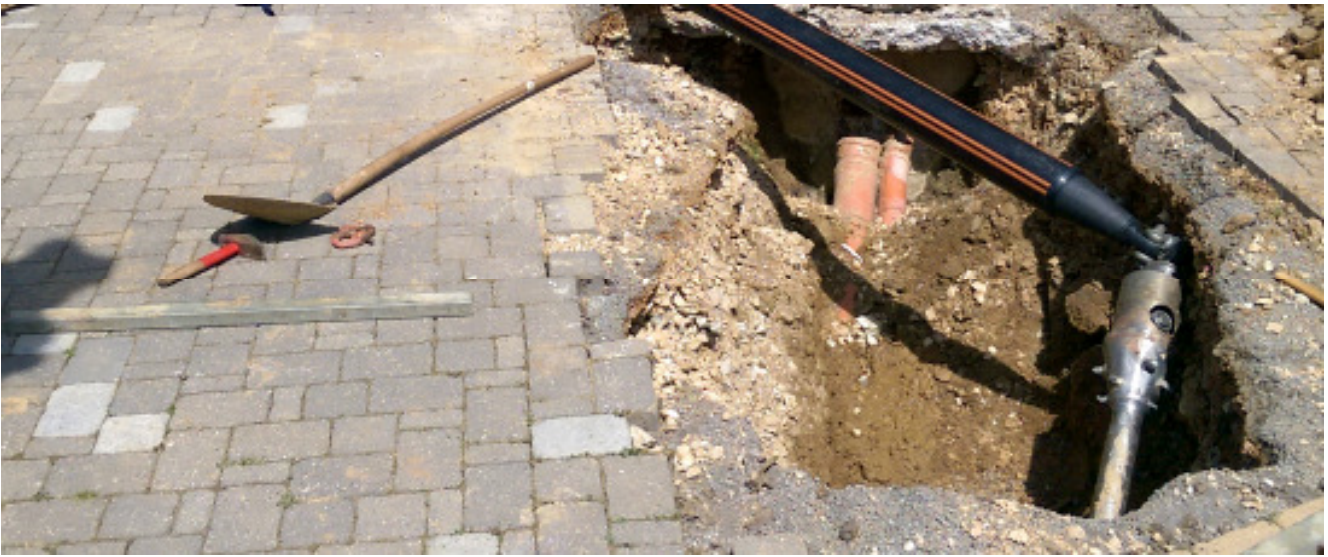
Pic. 4: After the successful pilot bore the product pipe HDPE OD 160 mm was directly pulled in. The picture above shows the backreamer \varnothing 215 mm with connected pipe just before beginning of backreaming with simultaneous pipe pull-in.
