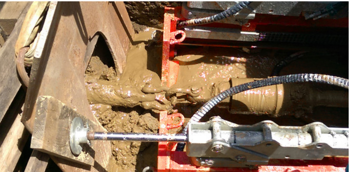
Pic. 5: The pit-launched-HDD-rig TERRA-JET TJ 3008 ES is designed in the way, that after pipe pulling-in the backreaming and towing tools can be towed into the rig itself. As a result starting pits with minimal pit length can be trenced and at the same time it is ensured that pipes can be pulled out of the ground sufficiently. Additionally that enables an easier removal of the tools after the job is done.
