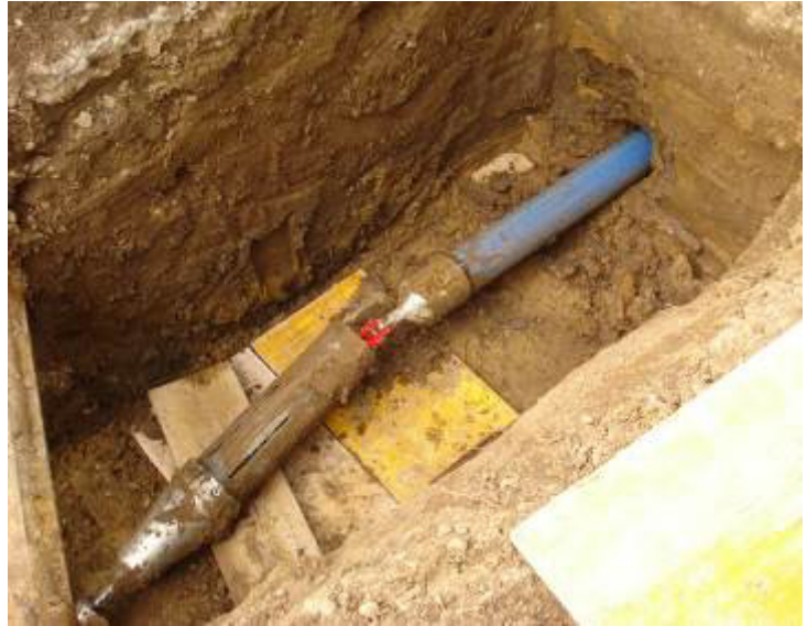
The cable burster was moved backwards in the machine pit, so that the expander cone and the new pipe can be disassembled. The new pipe can be connected to the fresh water system.
